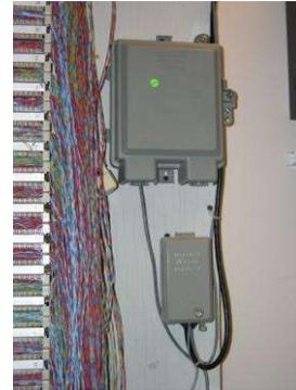
All components in the Telephone Switch Room are connected to a dedicated uninterruptible power supply (UPS) and then to the building's Emergency Power Circuit. In the event of the loss of public utility electric service, the UPS initially carries the load until the new MOC diesel fueled emergency generator with an automatic transfer switch supplies power to the telephone switch and connected components.
