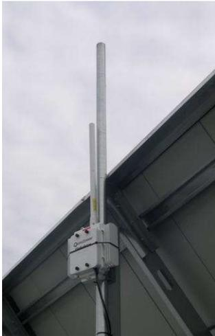
Once the SRAU was secured to the mast, cabling from the SRAU was run through a "roof penetration" to the Telephone Switch Room and connected to the satellite phone interface. Standard CAT5 wire connects the interface to the "punch block" and the dedicated telephone line. The PBX Switch was then programmed to identify the individual telephone extensions that have access to the SRAU.
